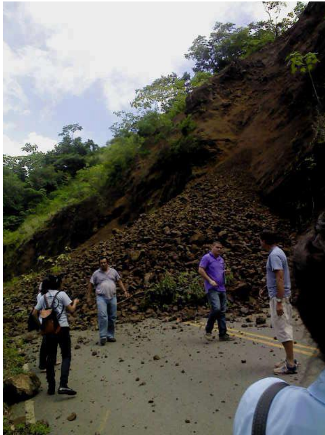
Landslide caused by the earthquake in Guanacaste
