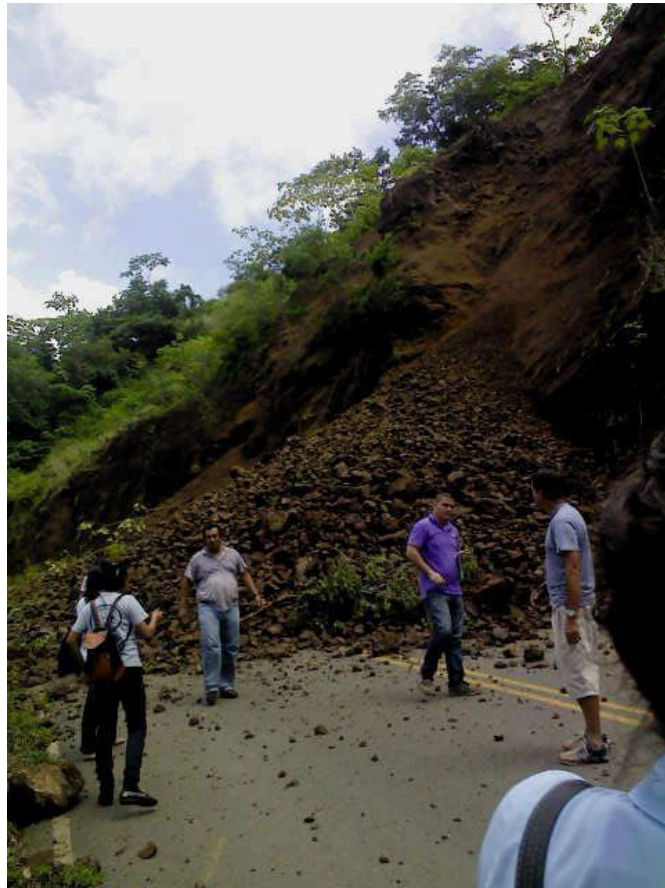
Landslide caused by the earthquake in Guanacaste
